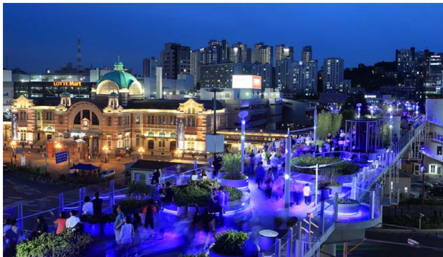
Following the example of the New York Highline, the former Seoul highway overpass was transformed into an approx. 1 km long Skygarden, situated 17 m above street level.
